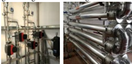
Fig. 4. Circulation pumps and secondary sludge-water HEX.
