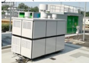
Fig. 3. First C50 SOFC Module.
