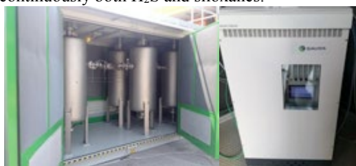
Fig. 2. Activated carbons reactors and online biogas monitoring system.
